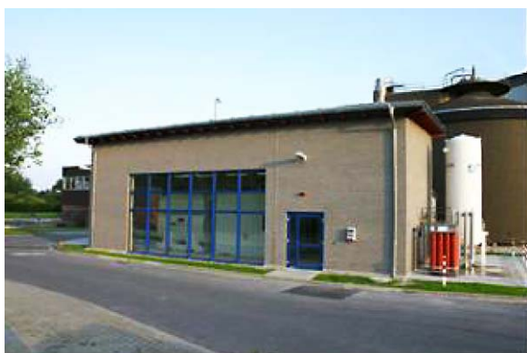
Fig. 1. Fuel cell building in Ahlen.
